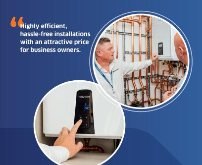
The system also included the high efficiency tankless NPE Water Heater, and NPE-A Cascade, which essentially links water heaters together, ensuring consistent hot water to multiple outlets, eliminating the risk of running out during periods of high demand.
