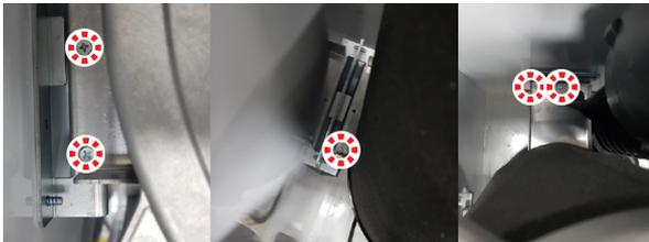
11. Remove the heat exchanger. The heat exchanger is heavy, so make sure to properly support it when removing it from the boiler.
