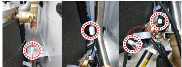
5. Open the drain valve of the lower return adapter to drain the boiler. Disconnect the air vent from the upper outlet adapter to drain faster.
