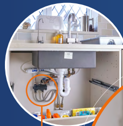
NaviCirc™ located under the kitchen sink.
