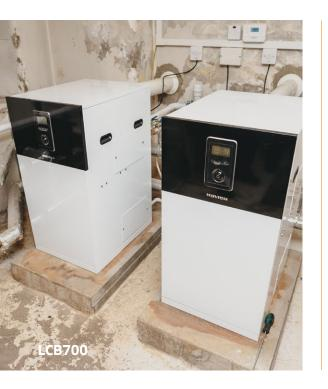
The original boiler was an antiquated cast iron atmospheric unit situated inside a small boiler house; this was replaced in August 2019 with a new, condensing system relocated in a separate workshop area. Navien became involved after the homeowner's son researched the options available online. The family contacted Steven McAllister, Area Sales Manager at Navien, who then offered guidance on the best options available.
